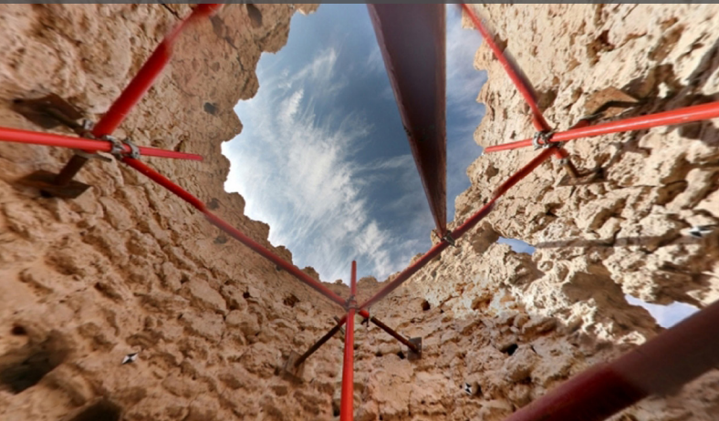
The tower heavily braced interior:
