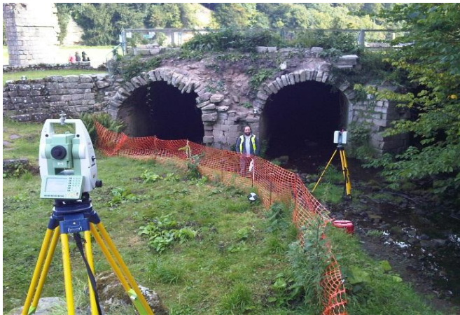
Surveying the tunnel entrances.
