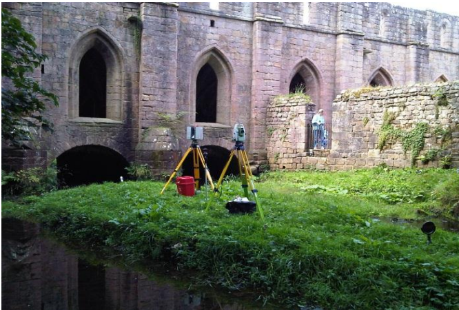
Use of a laser scanner to enhance traditional topographical detail.
